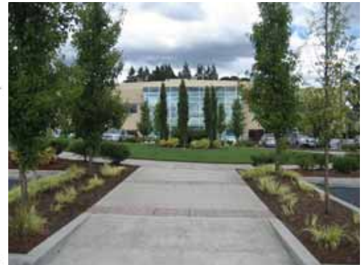
Example of well-defined building entrance
